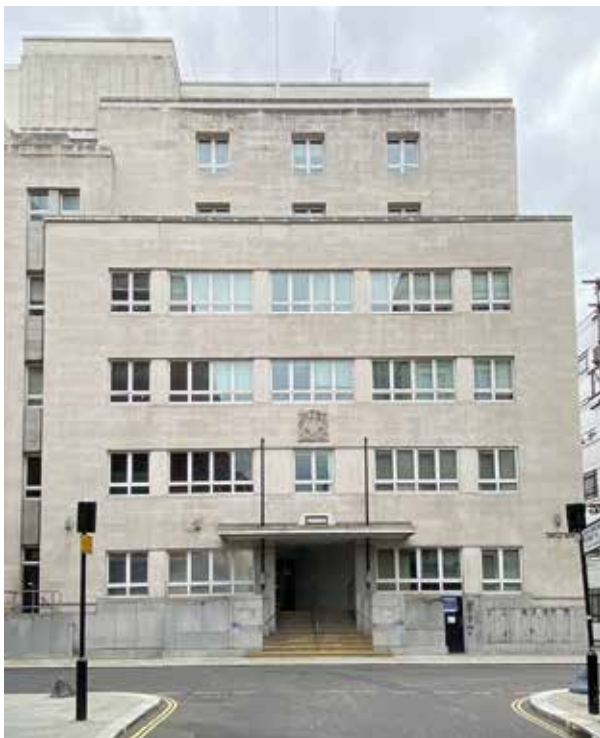
Existing view from New Burlington Street looking west
